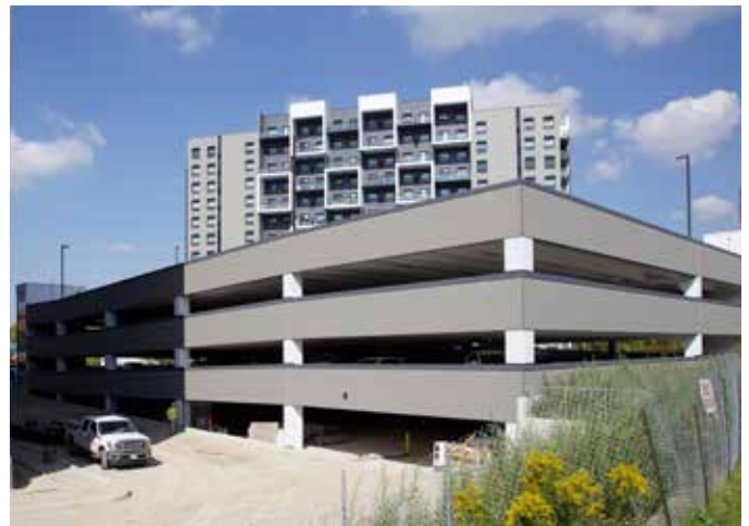
BELMONT PARKING GARAGE
